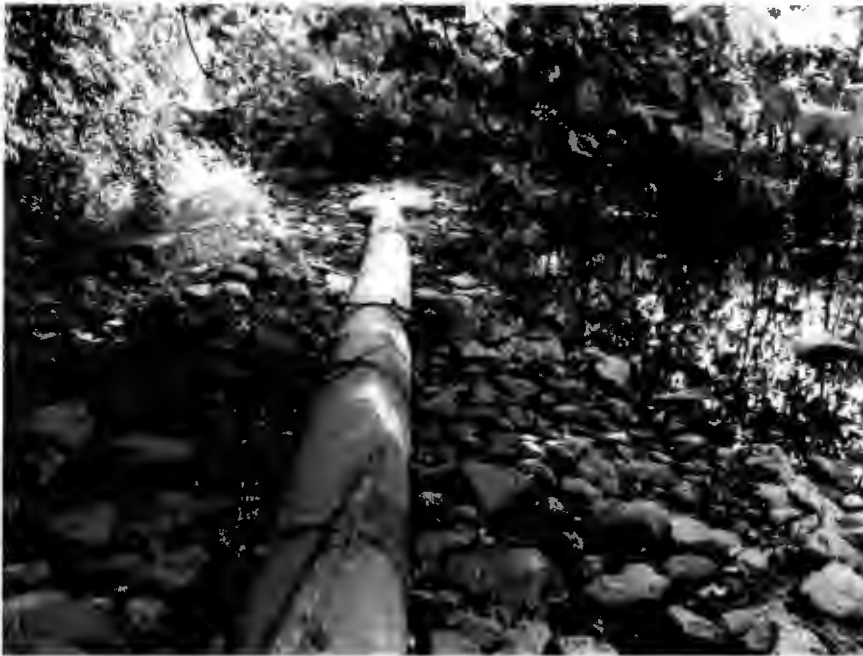
Picture shows the 18" diameter trunk sewer exposed in Wolf Creek (looking east).
