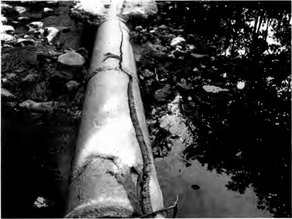
Picture shows detail of the cracked 18" diameter trunk sewer exposed in Wolf Creek (looking east).
