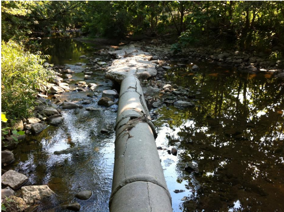
Picture shows cracked 18" diameter trunk sewer exposed in Wolf Creek (looking east).
