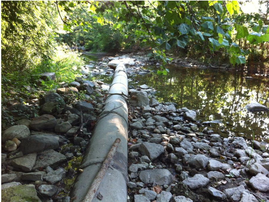
Picture shows the 18" diameter trunk sewer exposed in Wolf Creek (looking east).
